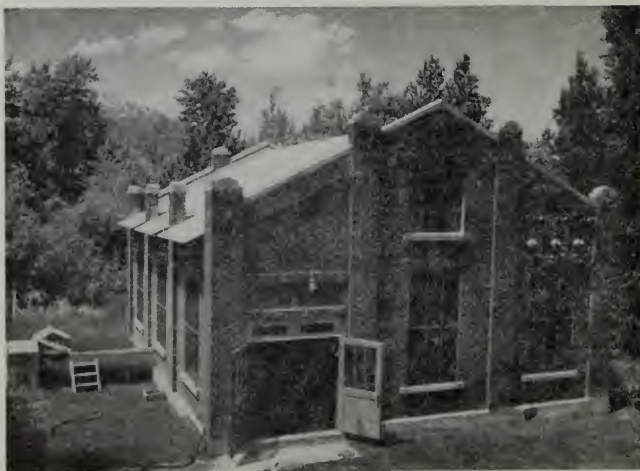
Joseph Generating Station constructed in 1923 by Inland Power & Light Company
